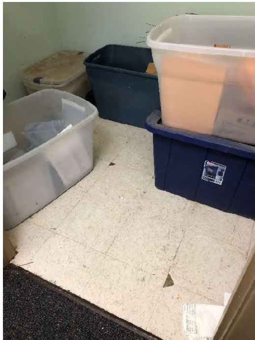
PHOTO 16: Shows the off-white, 12"x12", vinyl floor tile with gray splotches and yellow mastic sampled in the center storage room and HVAC closet (Samples VCT-05-50 through VCT-05-52). Testing of this material did not indicate the presence of asbestos.
