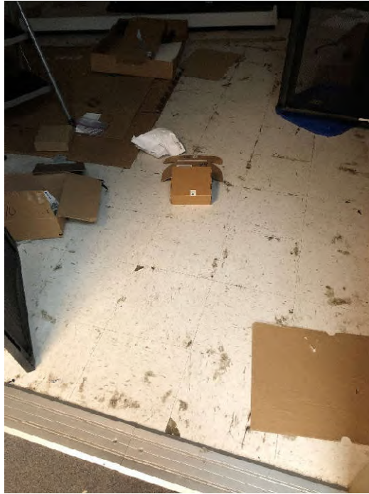
PHOTO 17: Shows the white, 12"x12", vinyl floor tile with beige splotches and yellow mastic sampled in the IT Server Room (Samples VCT-06-53 through VCT-06-55). Testing of this material did not indicate the presence of asbestos.
