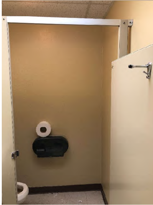
PHOTO 3: Shows the sheetrock wall system with wallpaper sampled in restrooms throughout the building (Samples SR-03-11 through SR-03-13). Testing of this material did not indicate the presence of asbestos.
