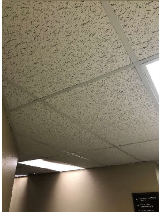
PHOTO 5: Shows the 2'x4', ceiling tile with pinhole and fissure pattern sampled throughout the building (Samples CT-01-17 through CT-01-19). Testing of this material did not indicate the presence of asbestos.
